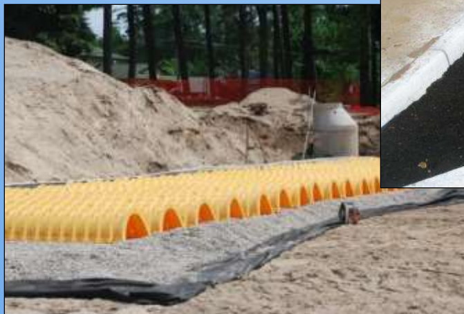
Underground infiltration trench installed at Bryant Park inTC
