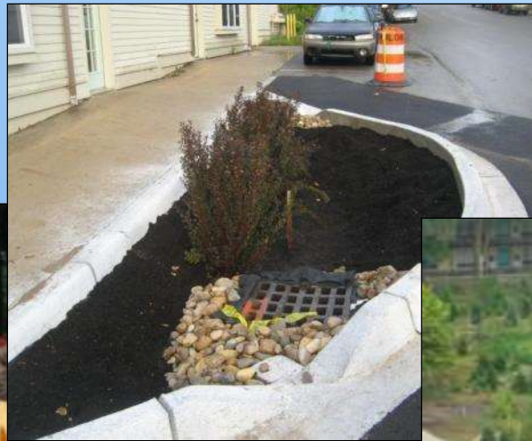
Rain garden in Suttons Bay
