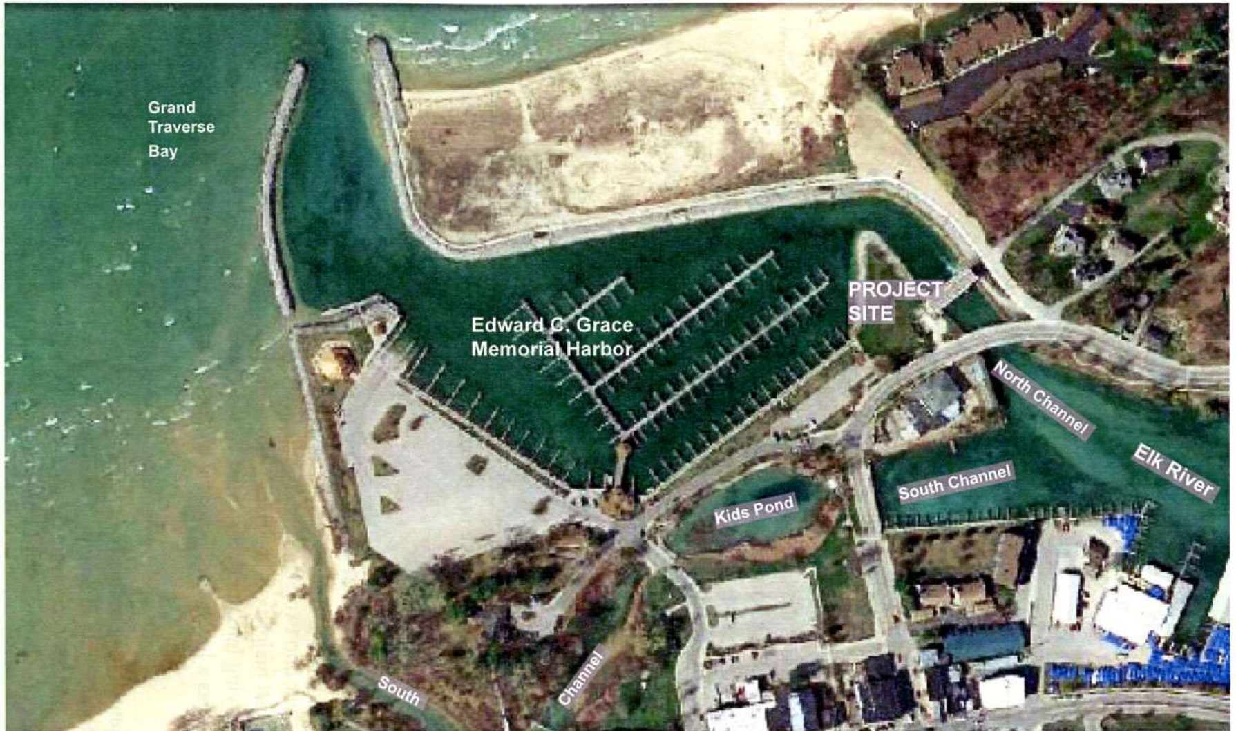
Aerial Showing the Configuration of Channels and Flow at Elk Rapids
