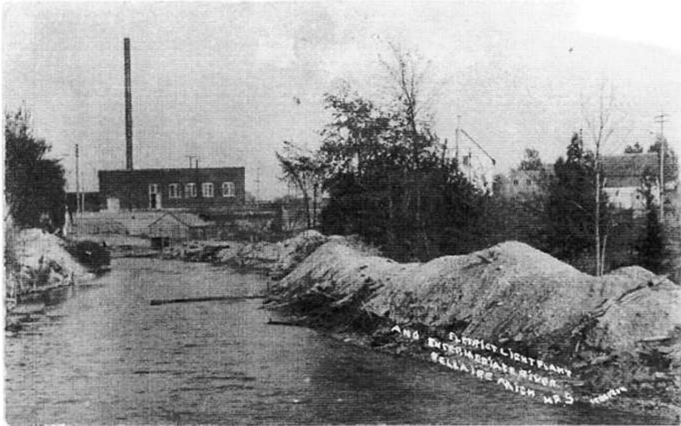
View Looking at Bridge Street from East Earthen Berms Show Dredging Activity on Intermediate River
