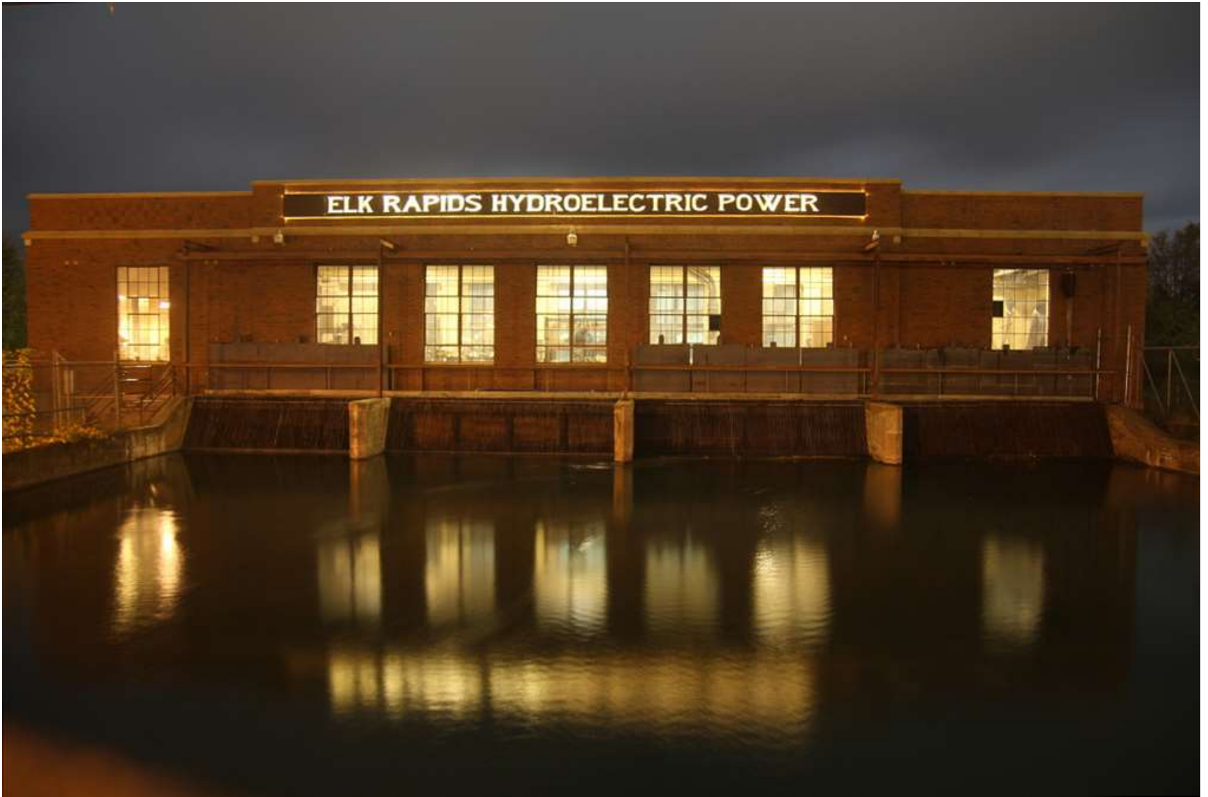
Continued Improvements on the Elk Rapids Dam
