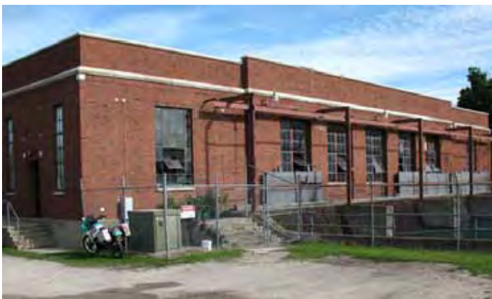
Photo 3 The Powerhouse Parking Area (Photo: ERHP 2009)
