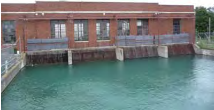
Photo 1 Front of Powerhouse and Headrace (Photo: ERHP 2009)
