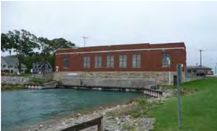
Photo 2 Back of Powerhouse and Tailrace (Photo: ERHP 2009)
