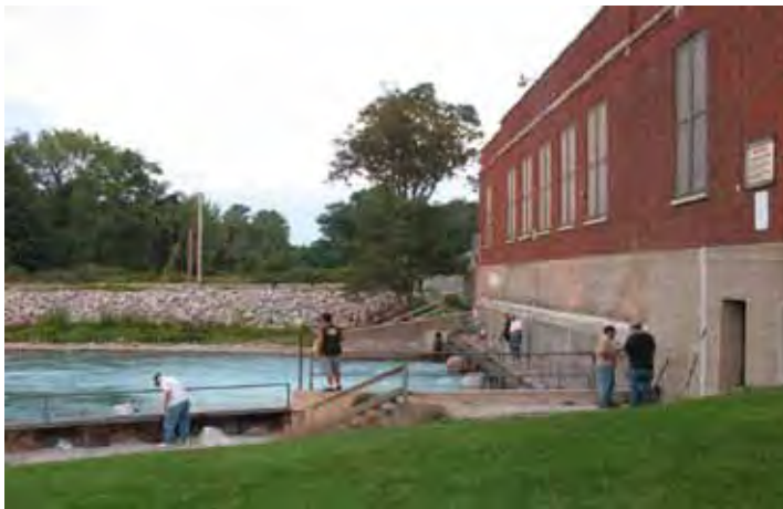
Photo 6 Fishermen Along the Back of the Powerhouse/dam (Photo: ERHP 2009) The back of the powerhouse is a popular fishing spot.
