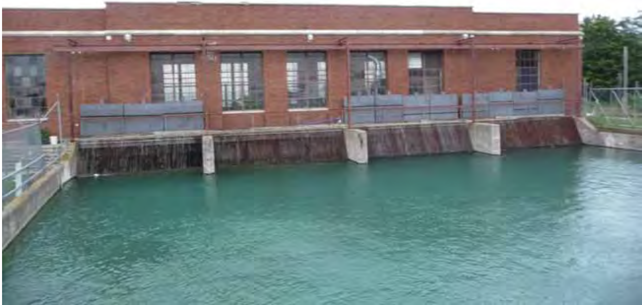
Photo A.1 Front of Powerhouse and Headrace (Photo: ERHP 2009) The two bays in the right of the photo contain the turbines.
