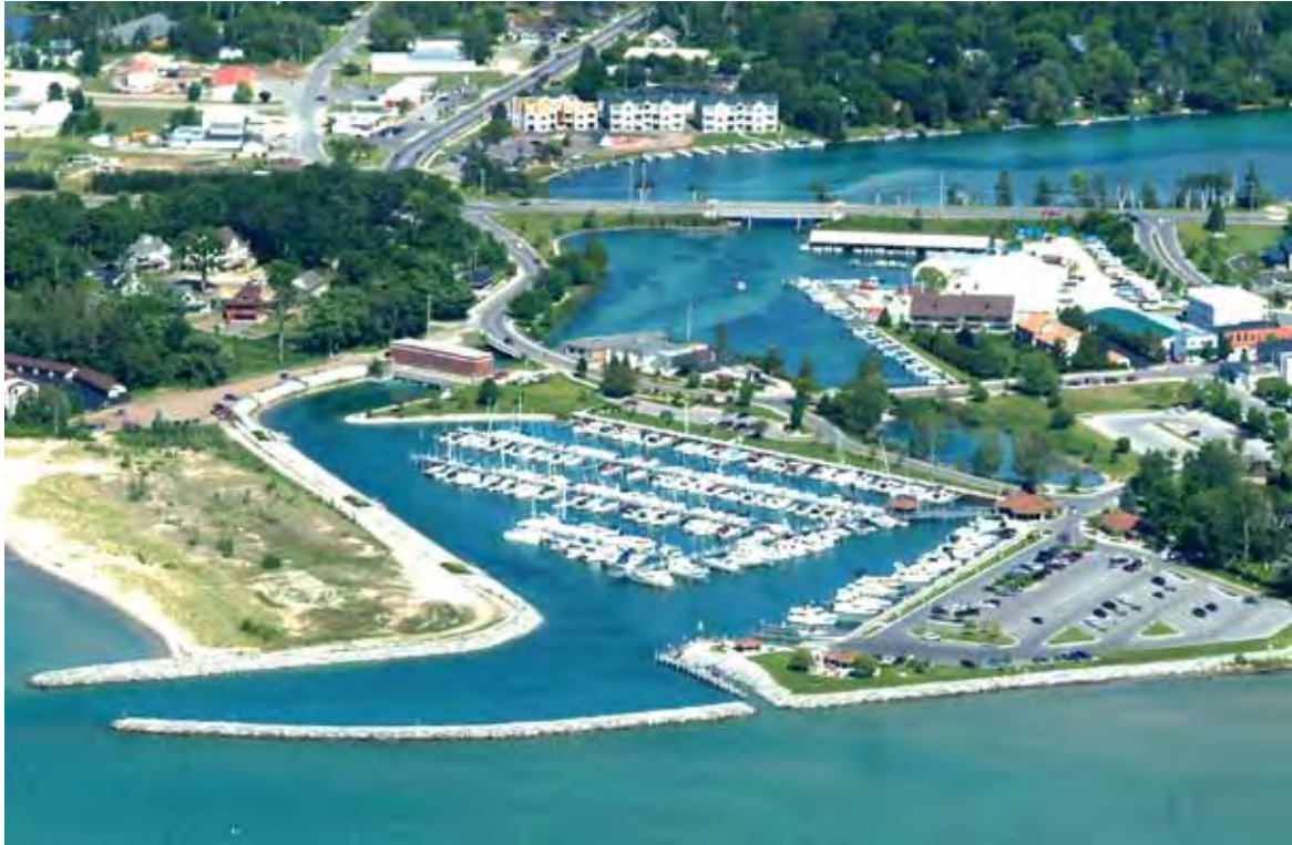
Photo 8.1 Aerial View of the Village of Elk Rapids (Photo: Jim Anderson 2005) The Project powerhouse can be seen spanning the river in the middle left, above Edward C. Grace Memorial Harbor. The village center continues off the right of the photo.
