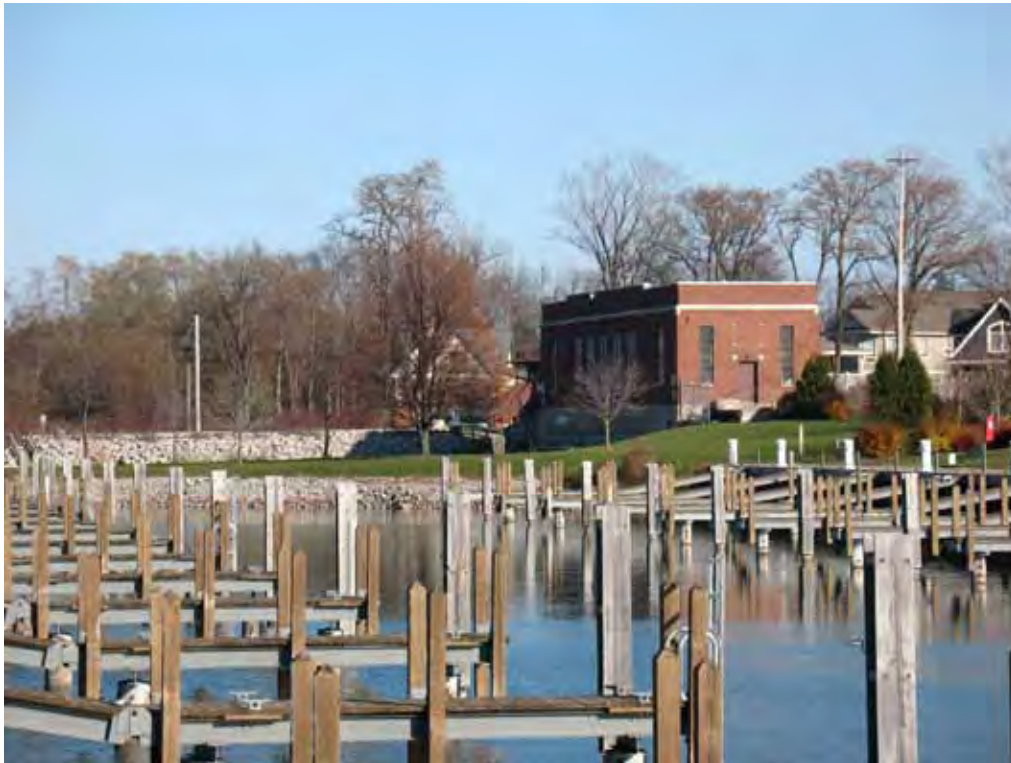
Photo 8.2 The Powerhouse in Autumn (Photo: ERHP 2009)
