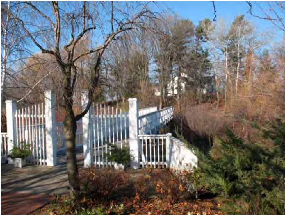
Photo 9.2 Island House Bridge (Photo: ERHP 2009)
