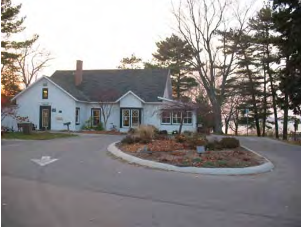
Photo 9.1 Island House (Photo: ERHP 2009)
