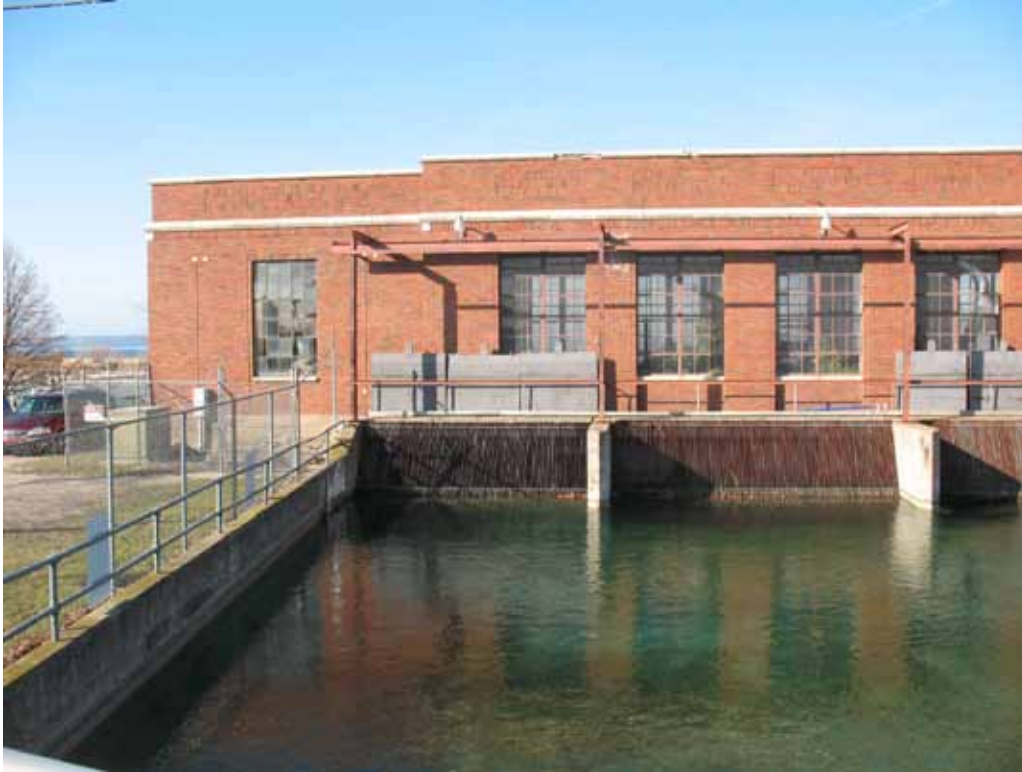
Photo E.12.1 Armored Shoreline at the Headrace (Photo: ERHP 2009)
