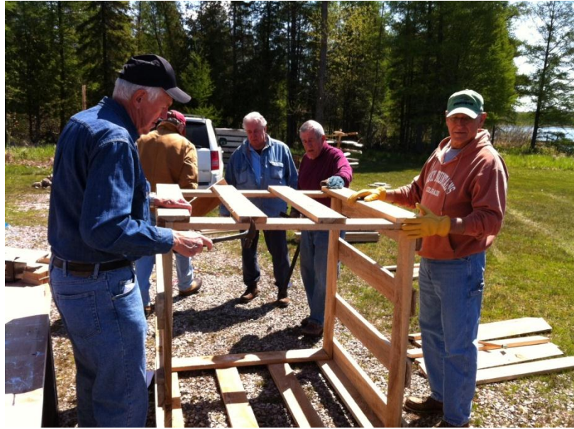
Figure 2. Construction of crate shelter
