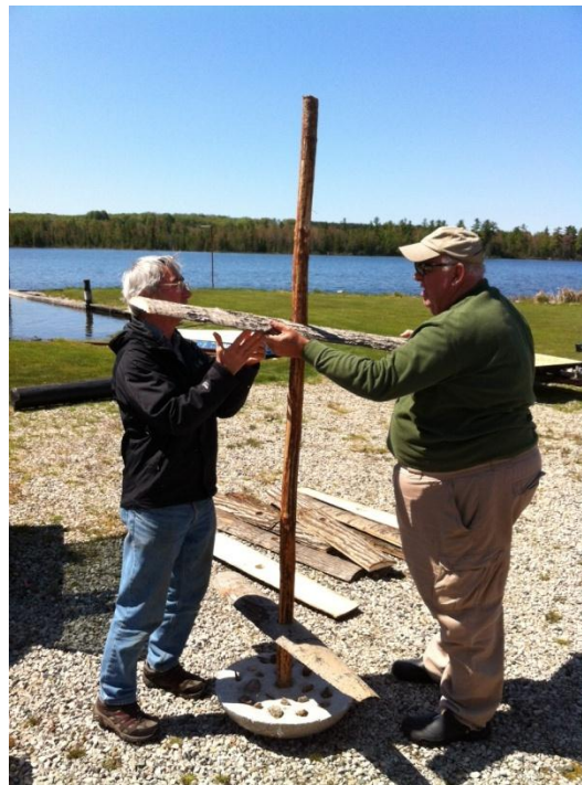
Figure 1. Construction of split log shelter
