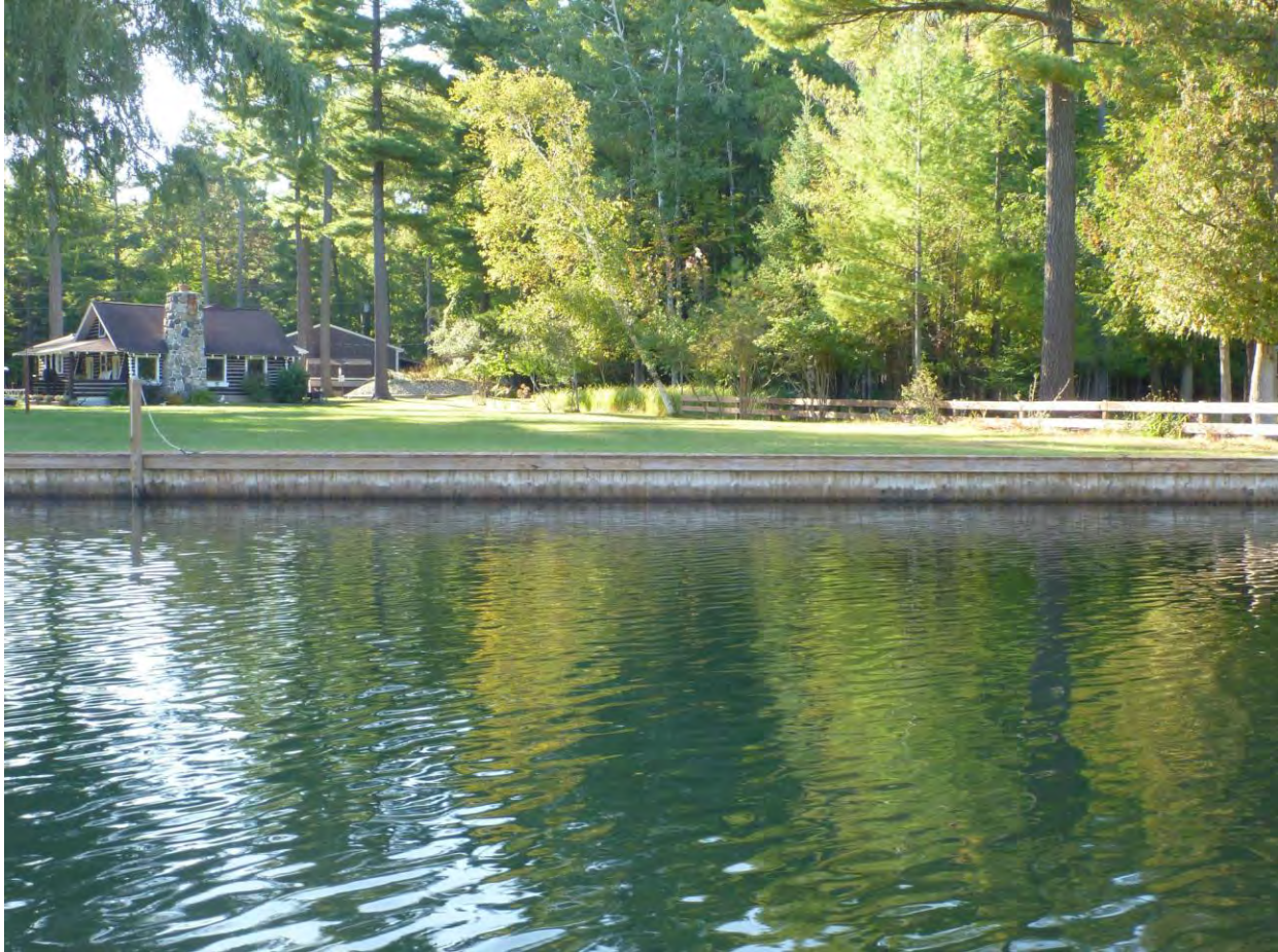
Figure 34. Image further downstream from Figure 33, in the middle Torch River. Visible is the completely armored bank of a wooden seawall.
