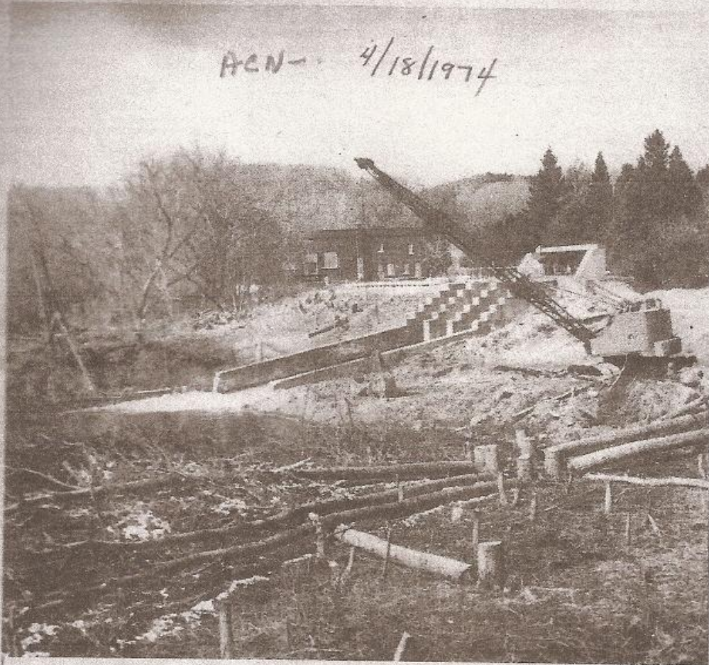
RECONSTRUCTION is well underway at the Intermediate River Dam in Bellaire. Work includes construction of a new Spillway as well as repair of the existing spillway structure. The old power house, seen in the background, will be removed as part of the overall improvement plans. John Arfel of Bellaire contracted to do the work.
