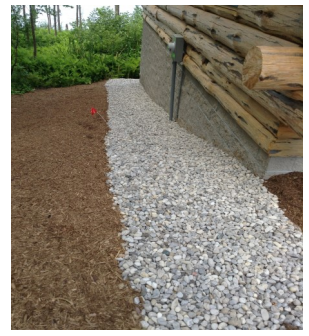
Rock filled trench at eave line
