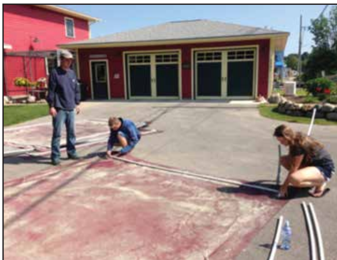
Assembling Benthic Barriers
