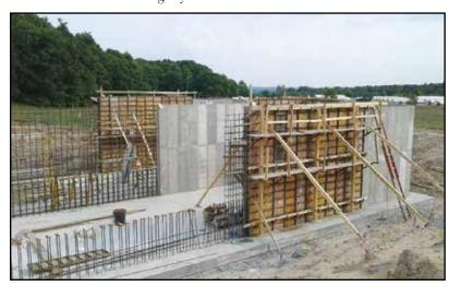
Poring the cement walls for two side-by-side 150,000-gallon storage tanks; each tank is 68 ft long, 23.5 ft wide, 14 ft high. Total volume of these two inground tanks is 44,744 cubic feet, which corresponds to 334,685 gallons.
