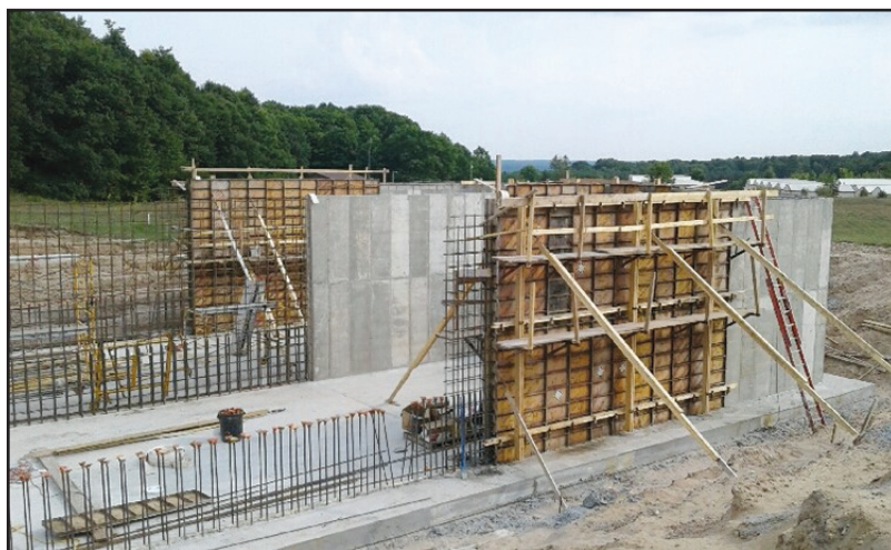
Poring the cement walls for two side-by-side 150,000-gallon storage tanks; each tank is 68 ft long, 23.5 ft wide, 14 ft high. Total volume of these two in-ground tanks is 44,744 cubic feet, which corresponds to 334,685 gallons.
