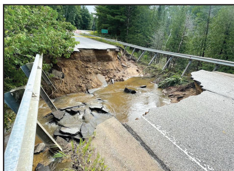
A culvert conveying Finch Creek under Alden Highway failed catastrophically during an extreme weather event in August of last year
